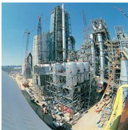
Union Bridge cement plant, USA
